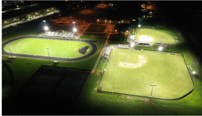
Marshall HS – Field Lighting
